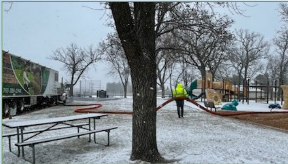
Wood chips being blown in at Community Park ( 176 yards).
