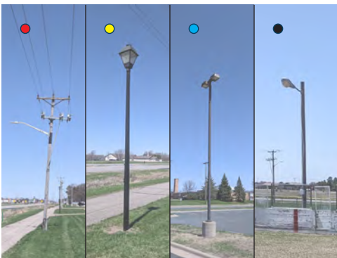
Existing Trail Lighting
