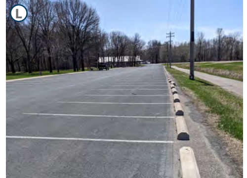
Existing Main West Parking Lot
