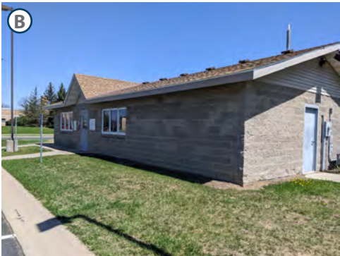
Existing Warming House
