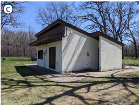
Existing Concessions and Restroom Structure
