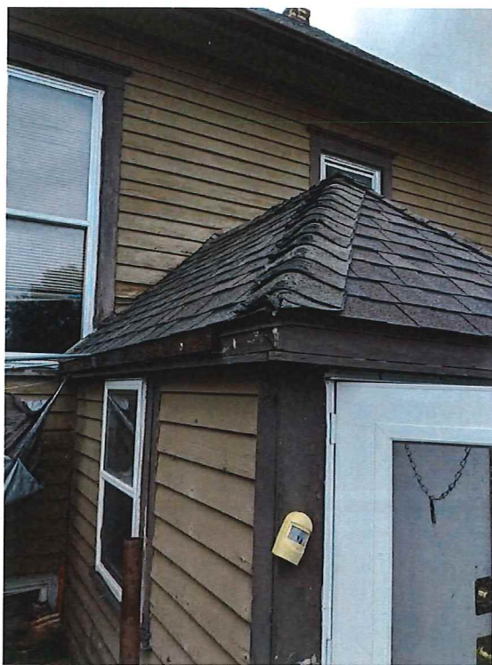
Photograph 11 - View of the east entry roofing.
