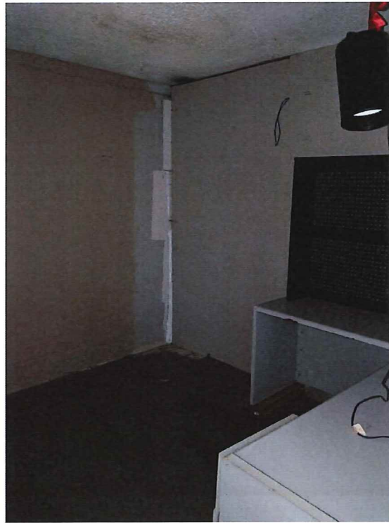
Photograph 58 - View of the office in the basement.
