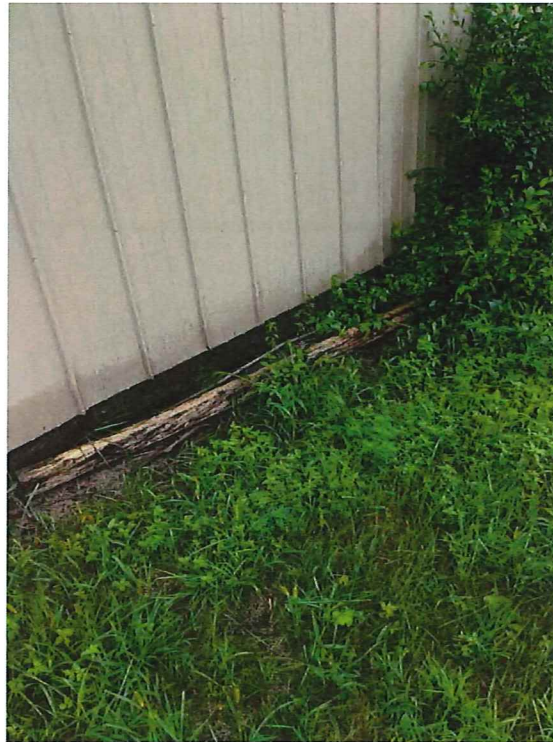
Photograph 32 - View of the timbers on the west side of the garage.
