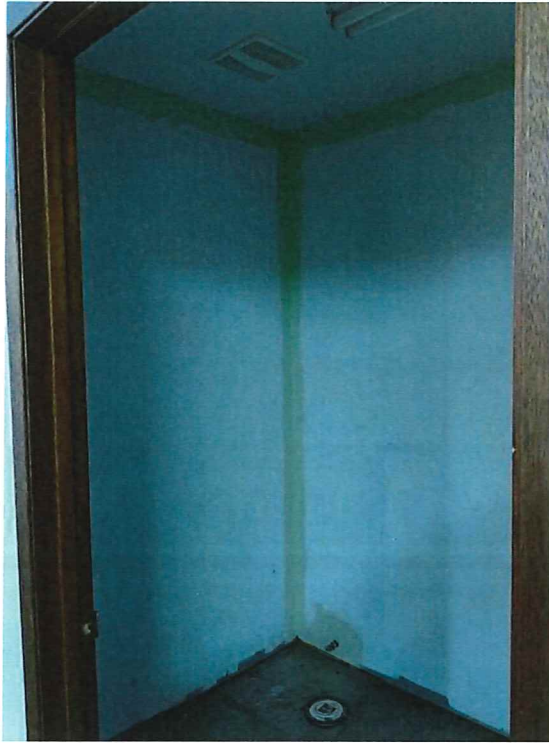
Photograph 25 - View of the storage room in the show room area.
