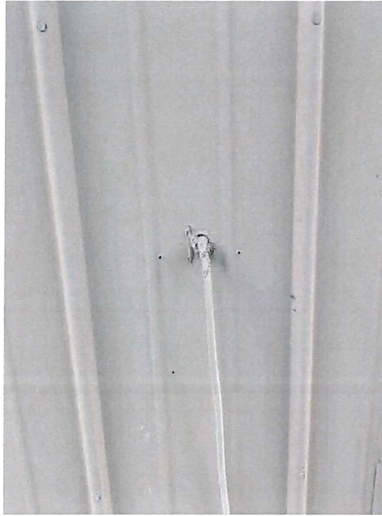
Photograph 31 - View of the pipe penetration caulking sample.
