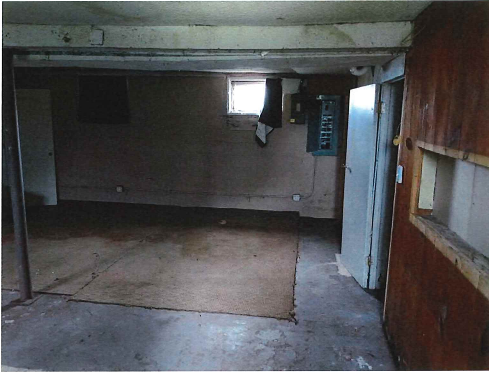
Photograph 57 - View of the basement.
