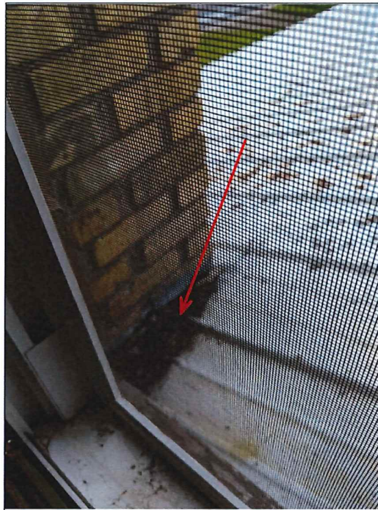
Photograph 52 - View of the chimney tar patch on the roof (Sample 10).
