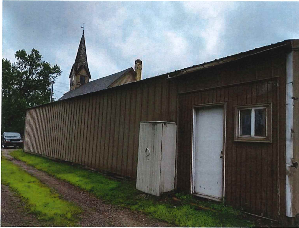
Photograph 13 - View of the east side facing southwest.
