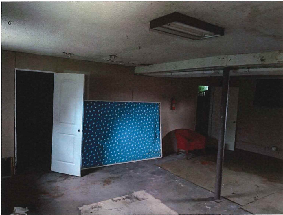
Photograph 56 - View of the basement.
