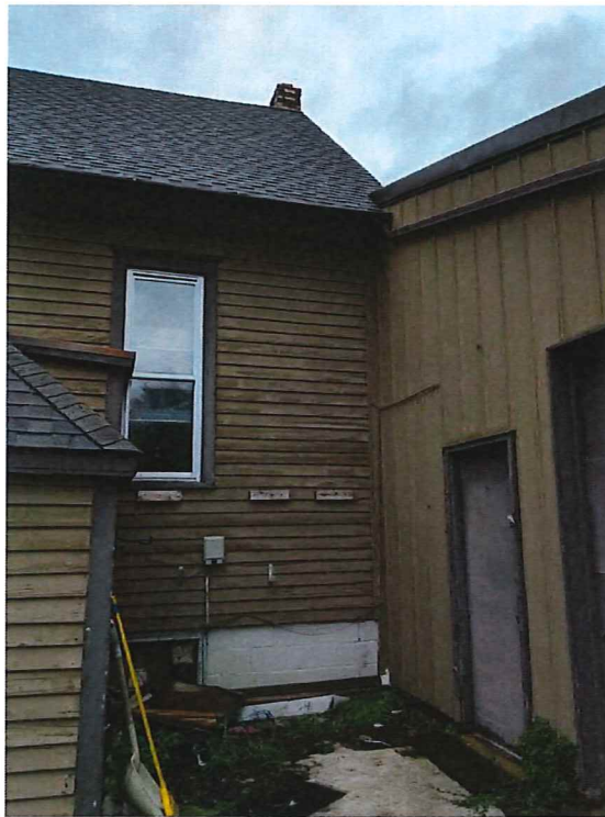
Photograph 6 - View of the east corner where the garage and house meet.
