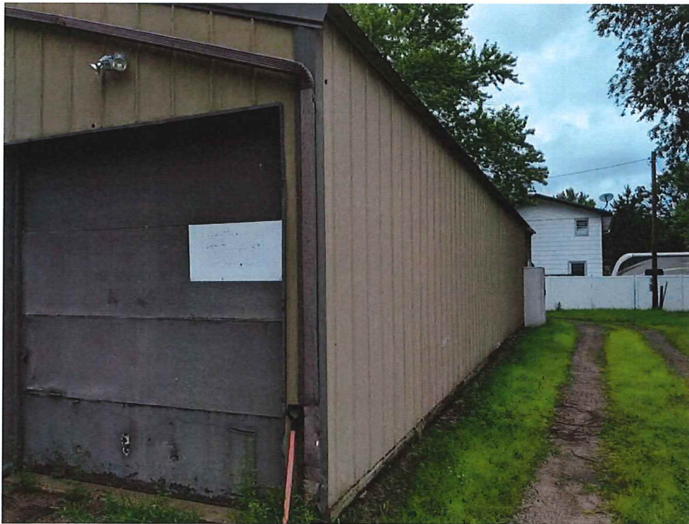
Photograph 8 - View of the east side of the garage.
