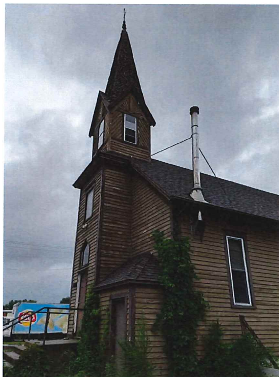
Photograph 2 - View of the east side of the church.
