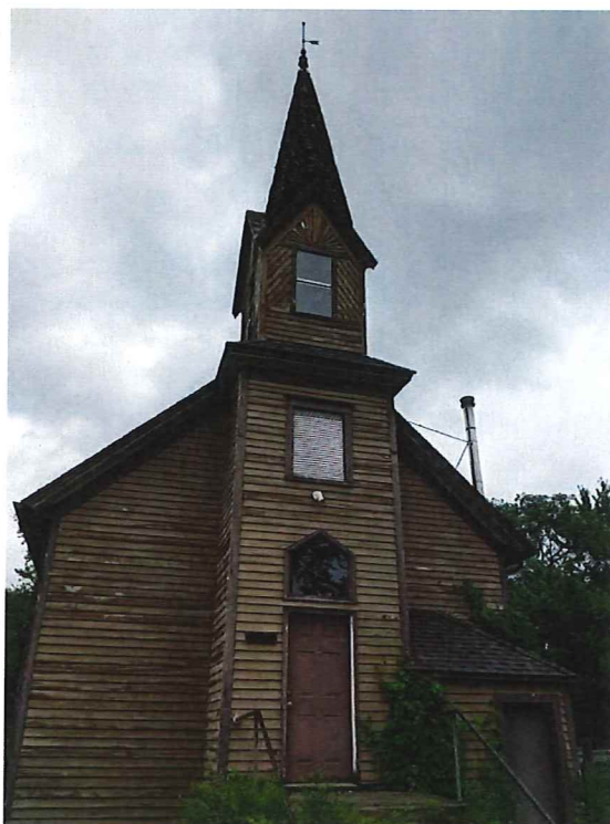
Photograph 1 - View of the south side of the church.
