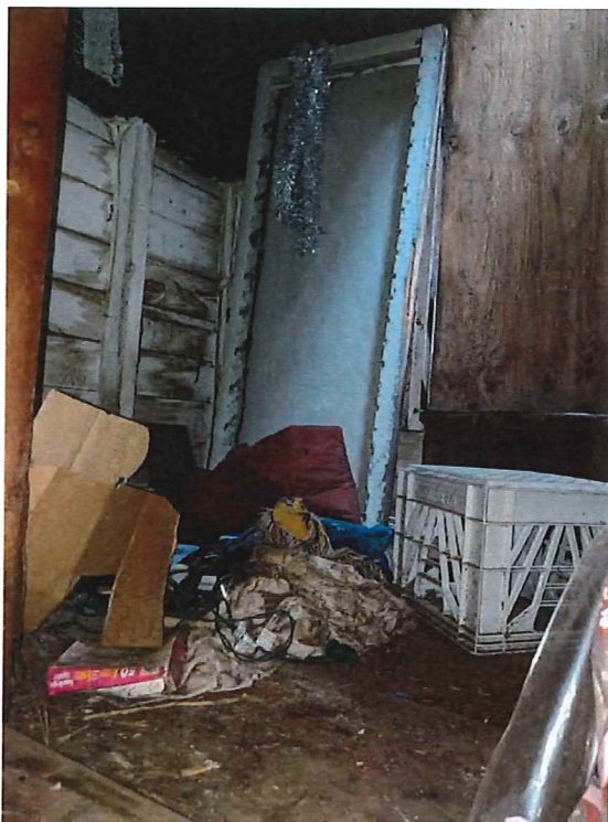
Photograph 61 - View of the steeple attic.
