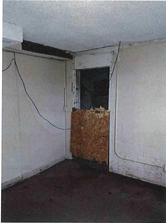
Photograph 59 - View of the bedroom in basement.
