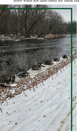
line away from the riverbank, making the bank less susceptible to erosion. The root wads collect sediment and debris to enhance the bank structure over time. They also provide structure for fish habitat.
