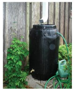
downspout. Rain barrels reduce the amount of stormwater runoff by collecting roof runoff and storing the rainwater for future use. By reducing stormwater runoff, we are also reducing the pollution that goes into our waterways.
